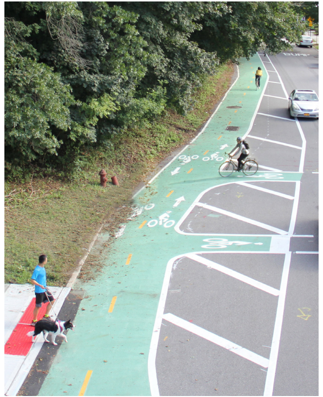
▲ This on-street path along 230th St in Queens provides access to Alley Pond Park and the Eastern Queens Greenway
